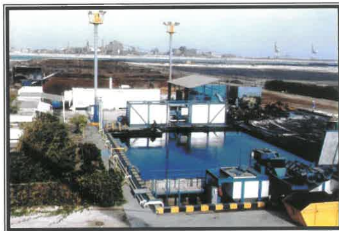
ASRY Dry Dock Reception Facility K. Bahrain
